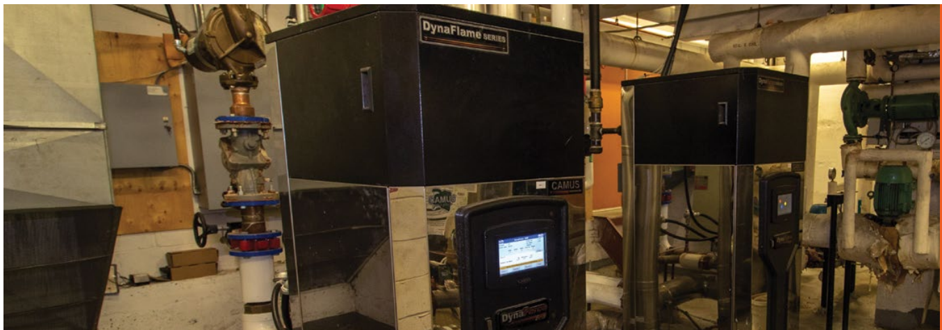
Figure 6: New boilers for space heating
