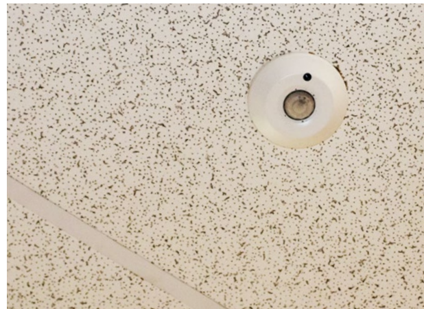
Figure 8: Motion sensor located in laundry room.
