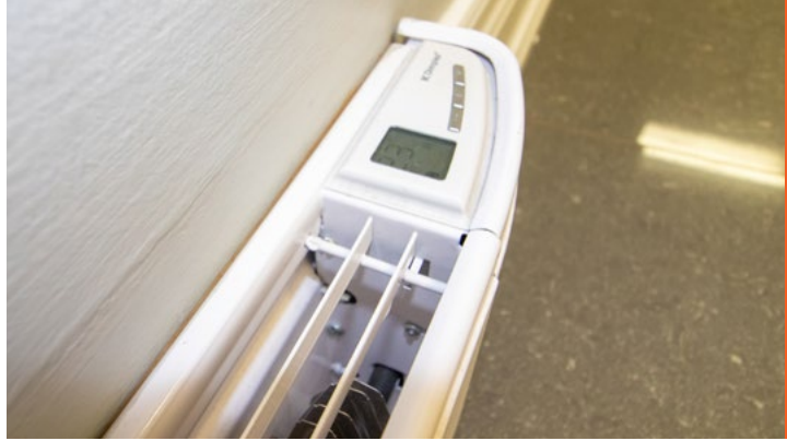
Figure 14: New electric baseboard
