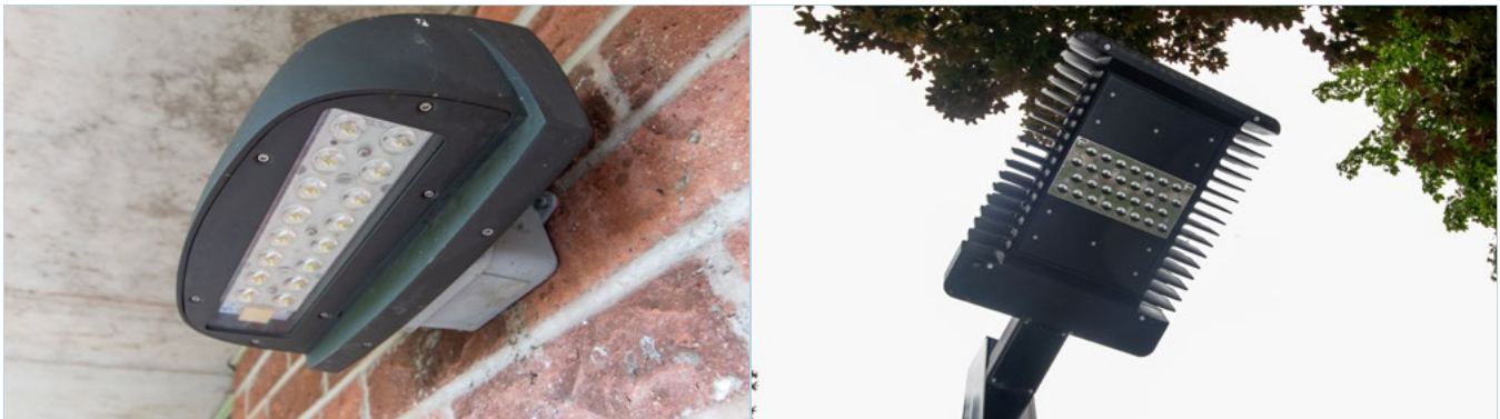
Figure 13: Examples of exterior LED lighting
