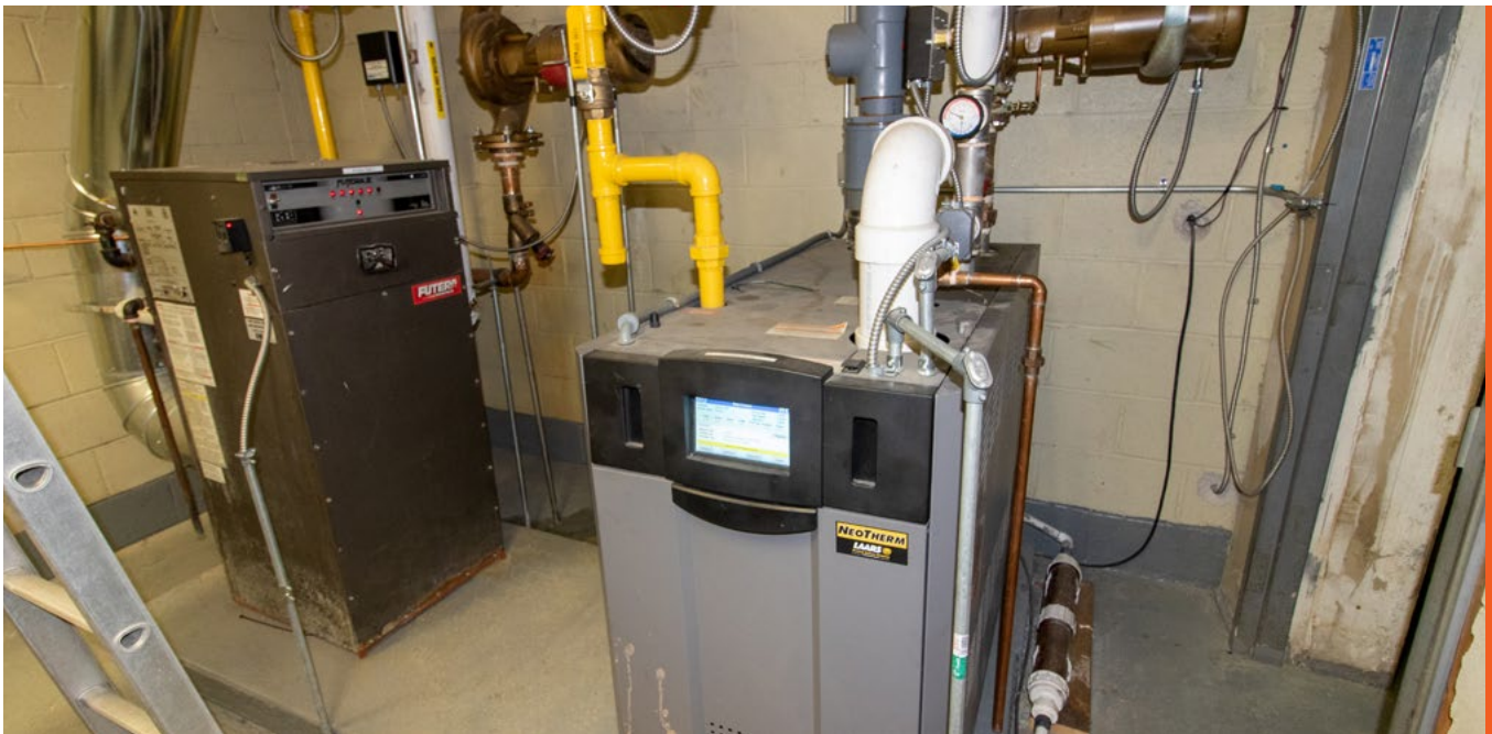
Figure 11: A Laars Neotherm boiler (right) was installed as the primary boiler
