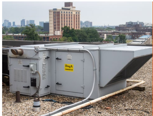
Figure 7: MAU on the roof
