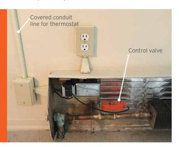
Figure 2. Typical control valve installation.
