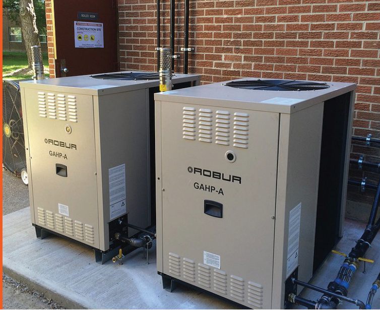
Two installed Robur GAHPs
