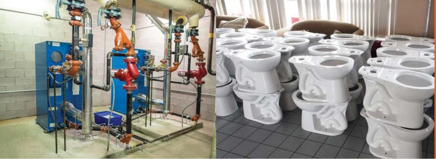
Left: two high efficiency boilers for domestic hot water; Right: low flow toilets awaiting installation.
