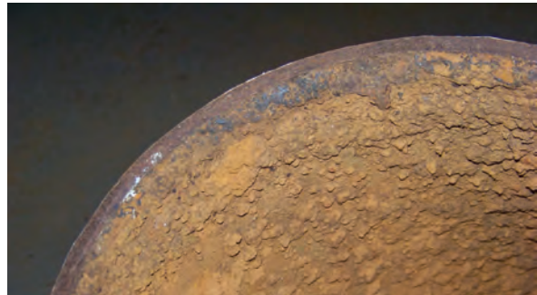
Pipe removed from untreated system
