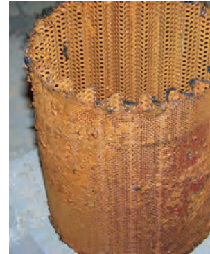
Suction diffuser screen from improperly maintained system
