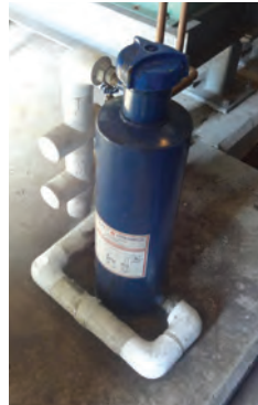
Chem-feeders must continuously contain the proper chemicals at the required levels
