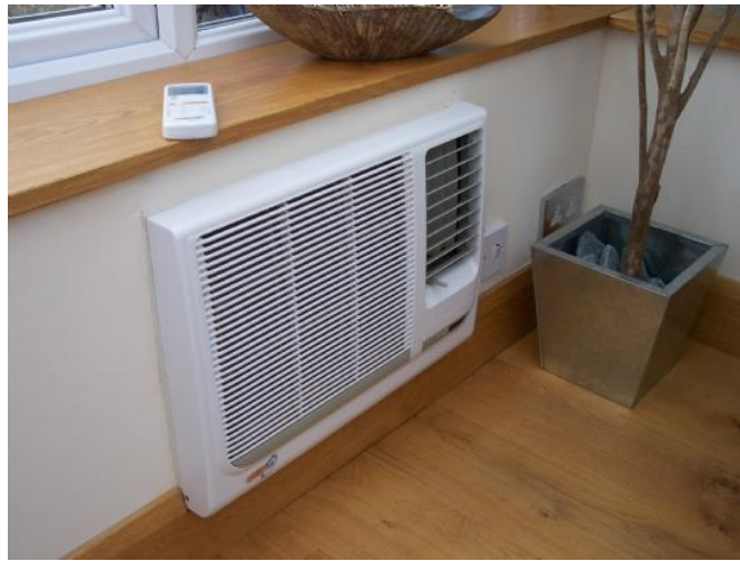
Figure 10: Single-Package Through-the-Wall System 16
