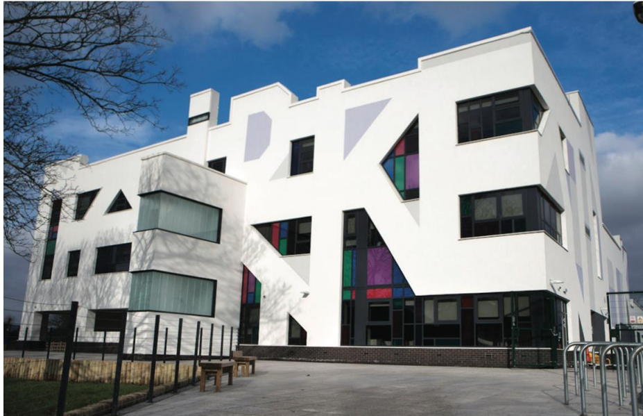
Figure 108: New Endike Primary School Building where 6 GWPL38 Gas Absorption Heat Pumps have been installed
