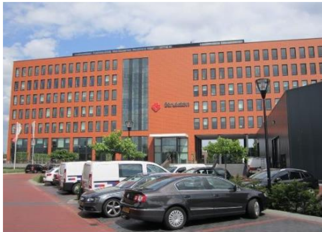
Figure 108: The Strukton Worksphere Office Building where 4 Aisin Toyota Gas Absorption Heat Pumps have been installed
