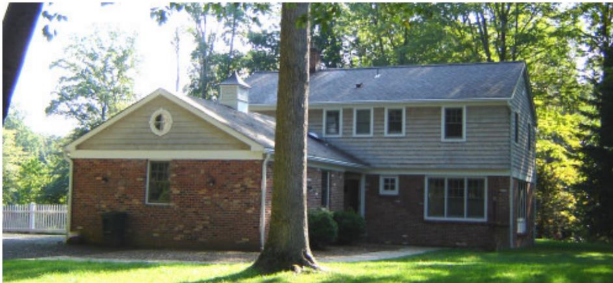
Figure 59: Test Site (Heat Pump is Located at the Back of the House)
