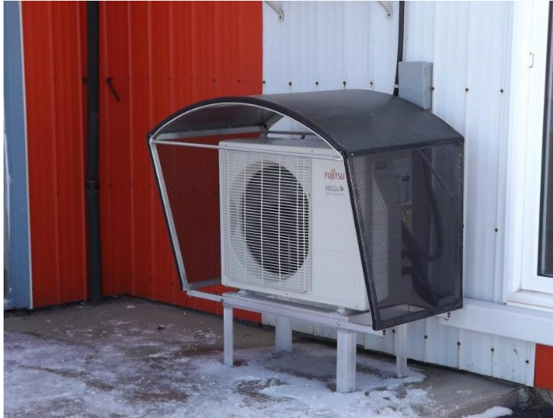
Figure 16: Heat Pump Cover 24
