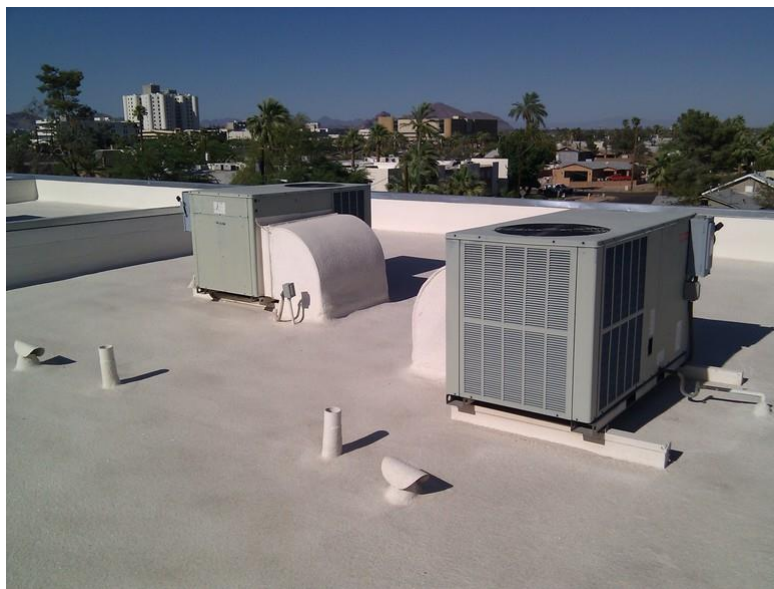
Figure 11: Single Package Rooftop System 17
