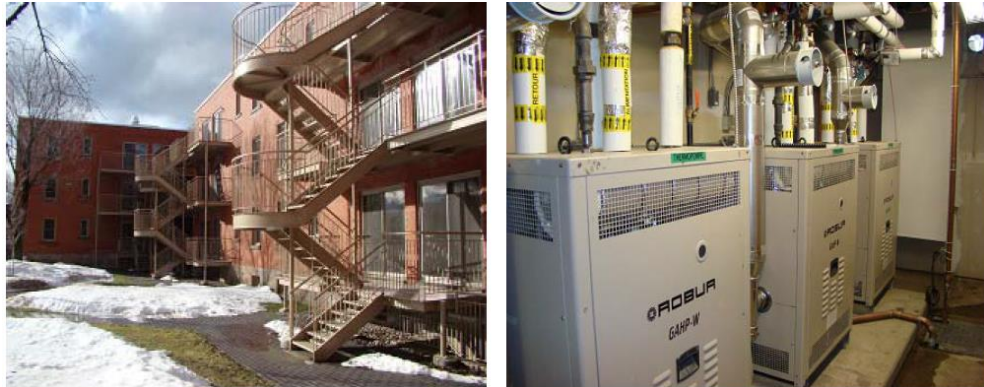
Figure 106: The Benny Farm Community and the 3 Installed Gas Absorption Water Source Heat Pumps
